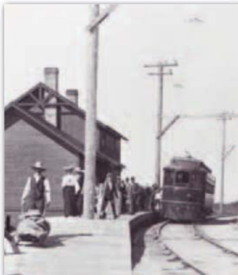
The BC Electric Railway tram, bound for Steveston from Vancouver, c. 1908. (VPL 2179)
